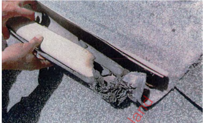
Photo 27: Shows cardboard Centre of a roll of membrane from 15 November 2019 fire reported to investigation team. Photo supplied by [REDACTED].
