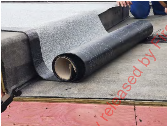
Photo 28: Cap Sheet torched on with residue roll left in gutter initially presenting little evidence of smouldering.
