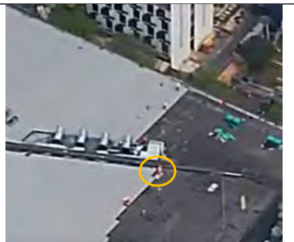
Photo 38: Roofer extends Cap Sheet to gutter while walking behind it. This would exclude the Cap Sheet being an unrolled section which could not be positioned if the worker was standing on it.
