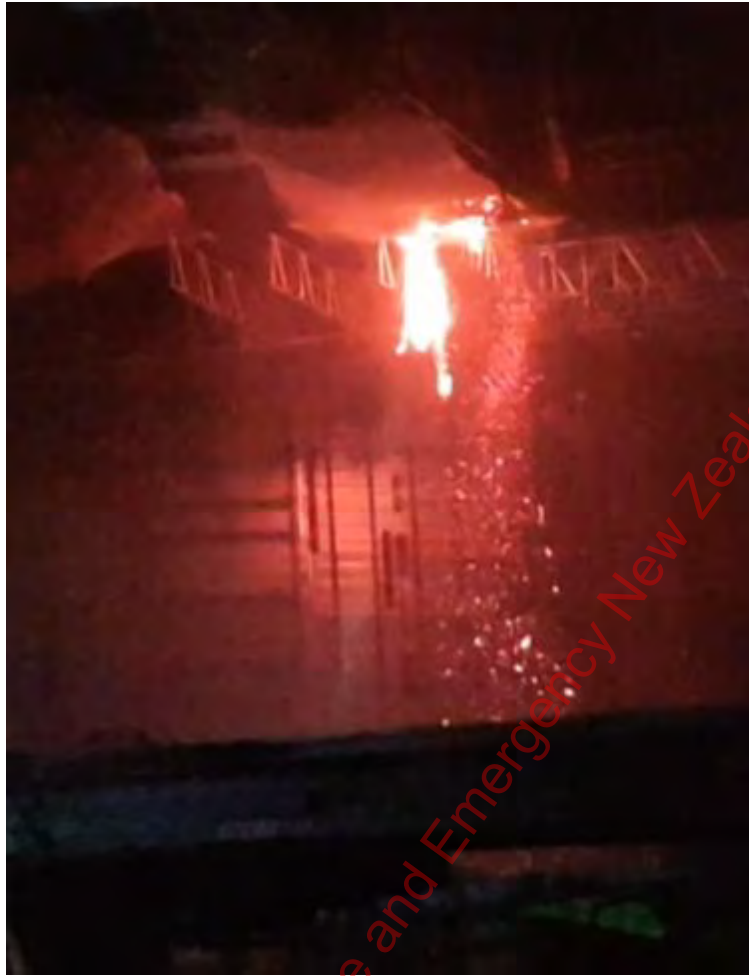
Photo 11: Burning elements within the ceiling construction collapsing on Day 2 providing a mechanism of fire spread to combustibles below.
