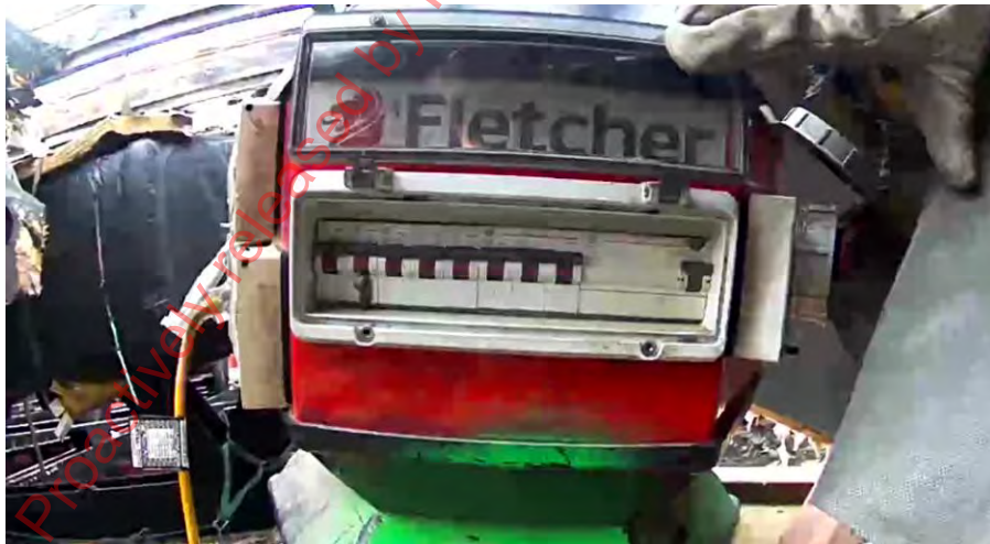
Photo 18: Power box with circuit breakers showing none had tripped.
