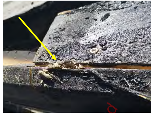
Photo 42: Example of roof on eastern side of Level 7, with residue sawdust in space between joints of plywood sheets (yellow arrow) extracted by investigators.
