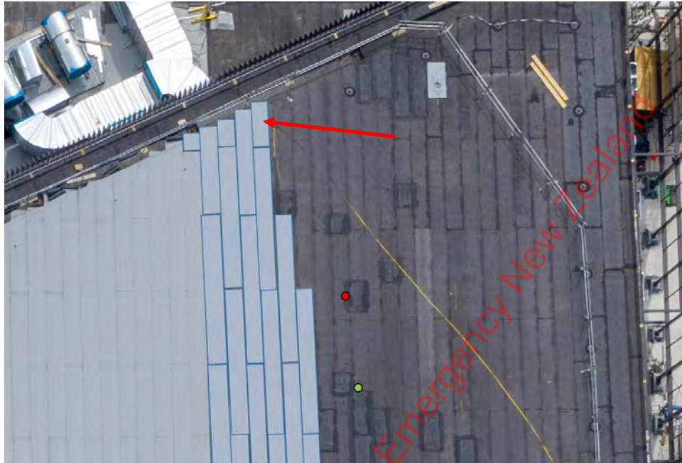
Photo 19: Shows position of the last short length of Cap Sheet laid to the gutter ~12:20 p.m. on 22 October 2019 (red arrow). Location of the 2 gas cylinders marked with red and green circles. Photo supplied by Fletcher Construction – additions by Fire and Emergency.
