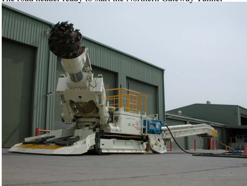
The road header ready to start the Northern Gateway Tunnel
