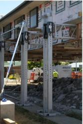
To prepare the house for lifting all bricks and flooring were removed. With the house now sitting on its brand new concrete foundation slab, the next step is to re-clad and complete internal repairs.
