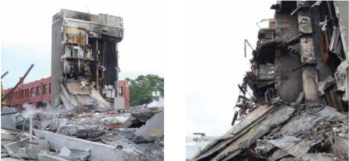
Figure 93: Figure 95 from the Hyland/Smith report showing the slabs lying against the north wall complex
