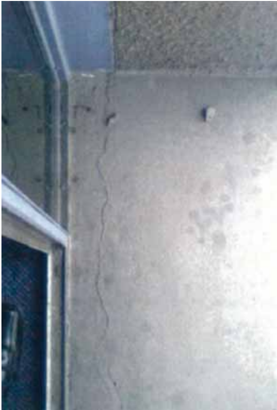
Figure 103: Cracking in south shear wall coupling beams (source: Leonard Pagan)
