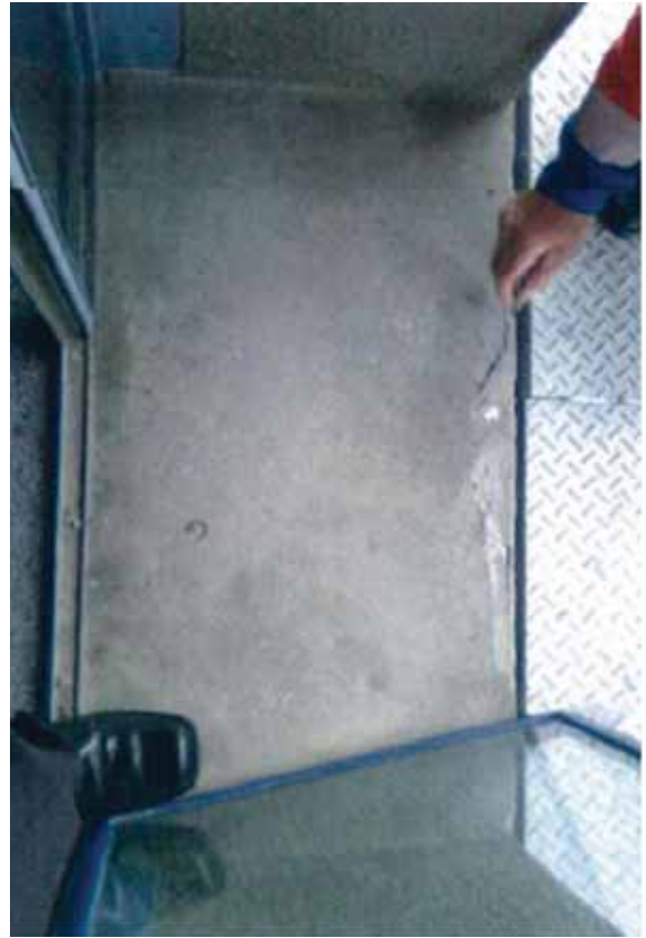
Figure 103: Cracking in south shear wall coupling beams (source: Leonard Pagan)
