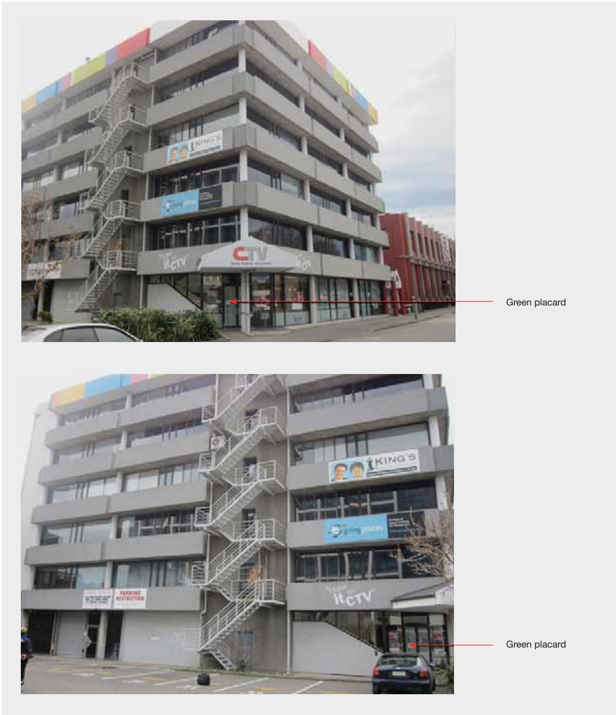
Figure 38: Photographs taken from respectively the south-east and the south of the CTV building by Richard Sullivan on 5 September 2010. The green placard can be seen on the main entrance door
