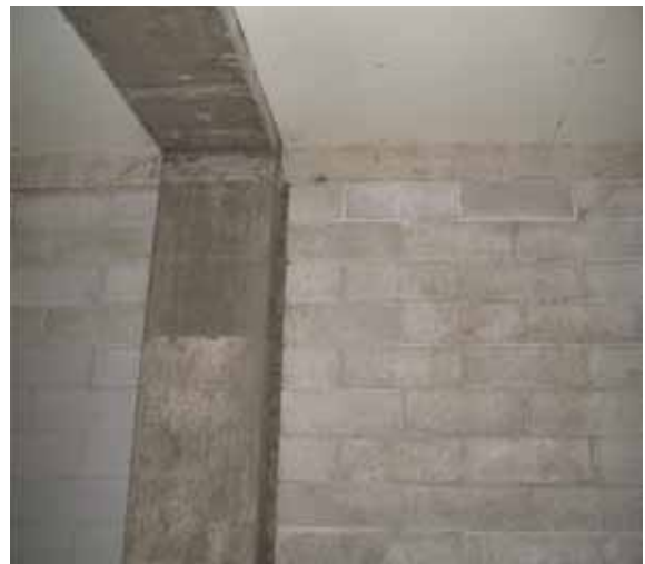
Figure 46: Western concrete block wall (source: David Coatsworth)
