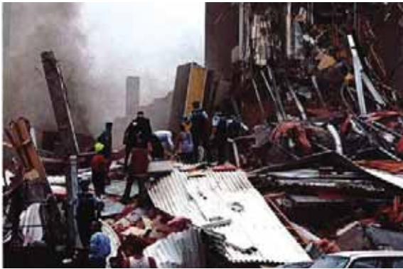
Figure 56: Photograph taken from the south-east corner of the CTV site approximately 30 minutes after the 22 February 2011 earthquake (source: Michael Williams)
