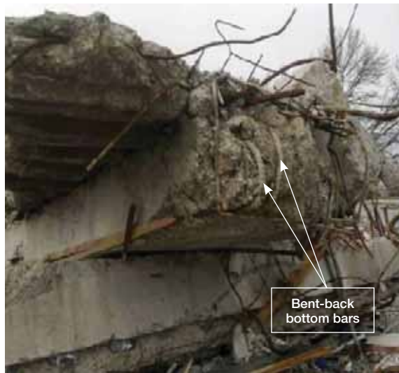
(b) End of beam with slab attached
