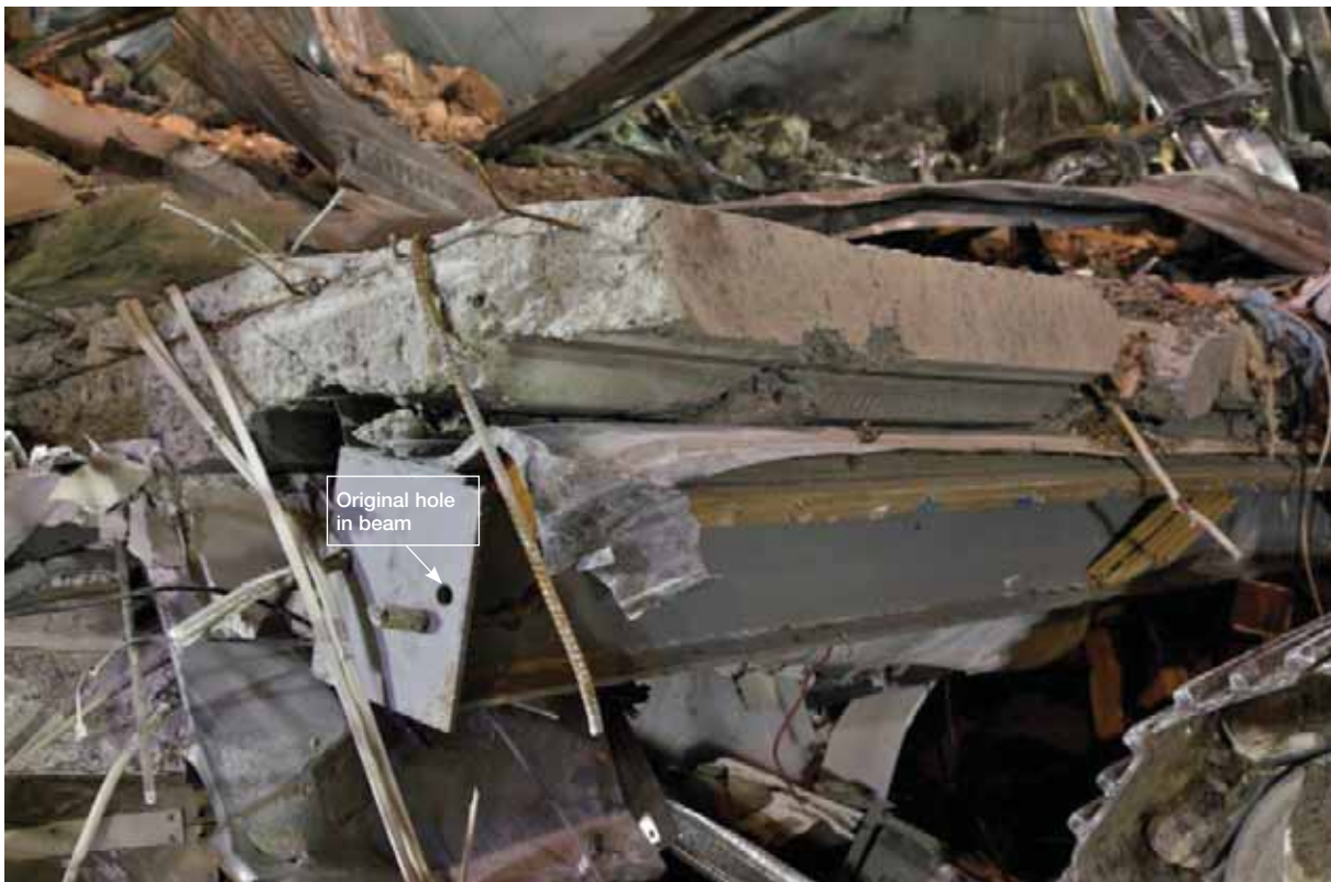
Figure 29: End of trimming beam
