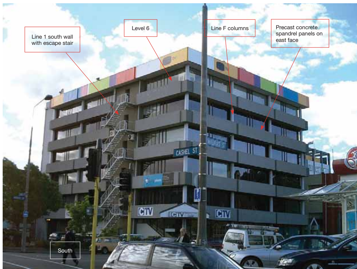
Figure 3: The CTV building in 2004. Shown in a photograph from the Hyland/Smith 1 report
