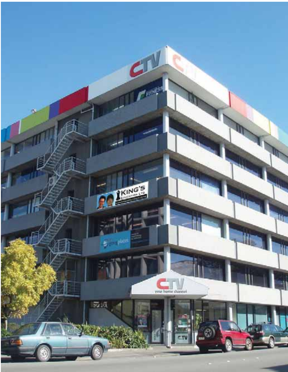
Figure 1: View of the south-east of the CTV building. Madras Street is in the foreground
