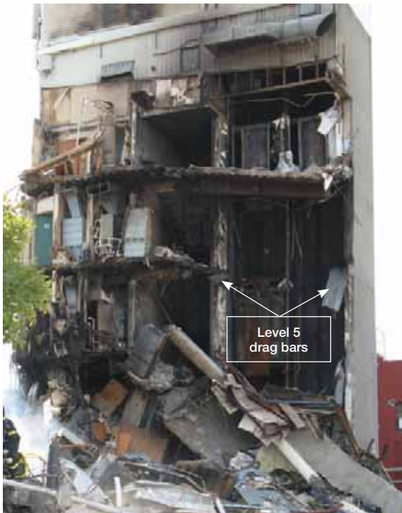
(a) The north wall complex after the collapse
