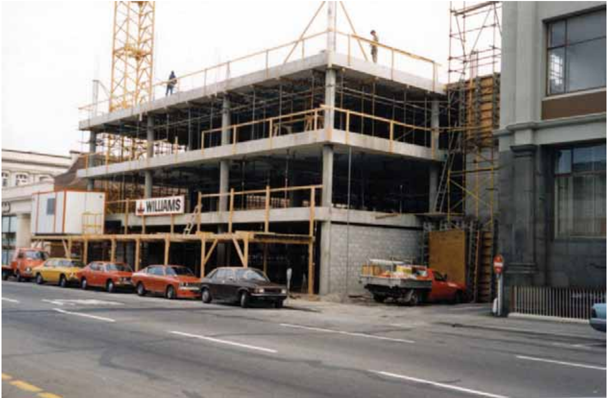
Figure 10: View from Madras Street before the installation of spandrel panels
