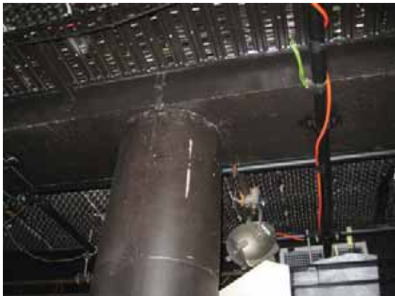
Figure 13: An interior column and beam on level 1
