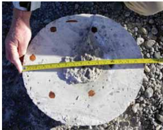
Figure 23: Slightly oval cross-section with poor control of reinforcement cover (source: Dr Robert Heywood)
