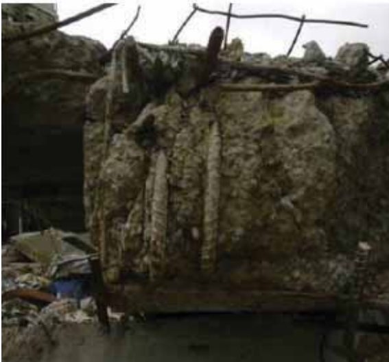
(a) Two H24 bars bent back into shell beam
