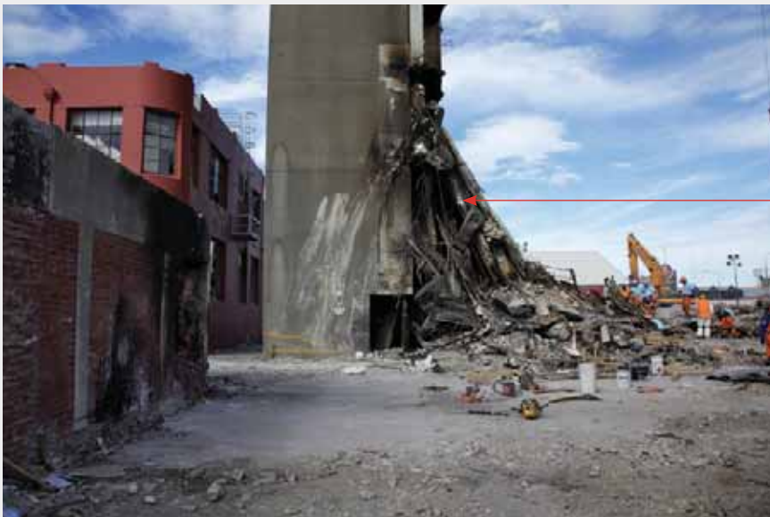
Figure 66(a): Western elevation of collapsed floor slabs leaning against north wall complex (source: Robert Heywood)
