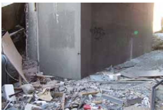
(a) Eastern elevation of wall complex (source: Graham Frost)
