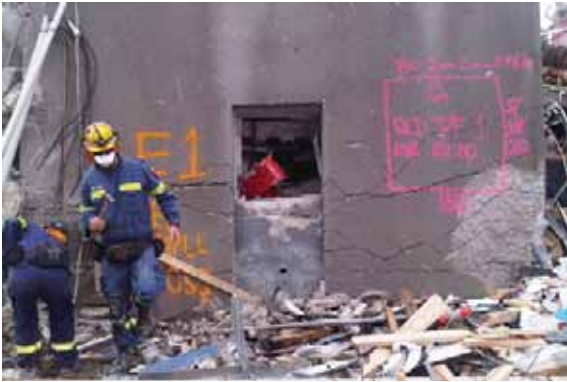
(b) Level 1 of the south shear wall (source: Graham Frost)
