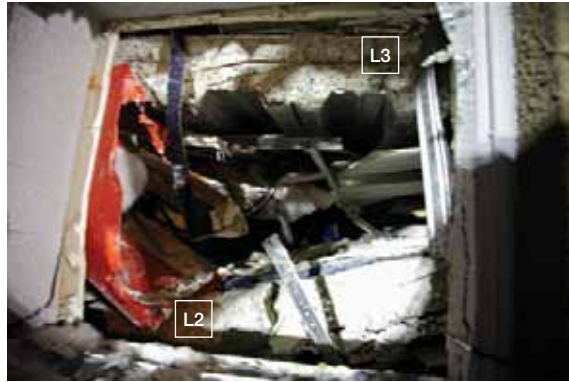
(c) Floor slab through level 1 door window (source: Robert Heywood)
