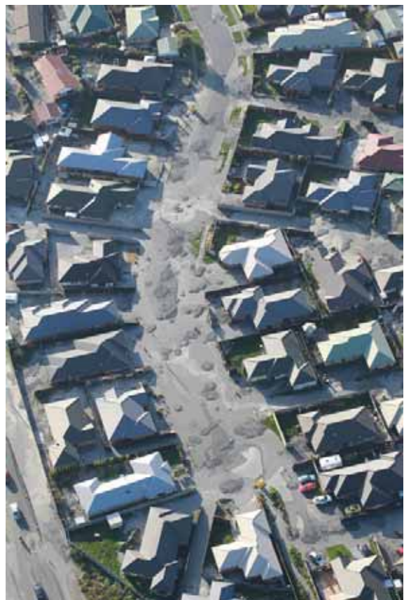
Figure 6: The eastern suburbs suffered repeatedly from liquefaction. This aerial photo shows a street in Bexley after the June 2011 aftershock (source: Fairfax Media/The Press)
