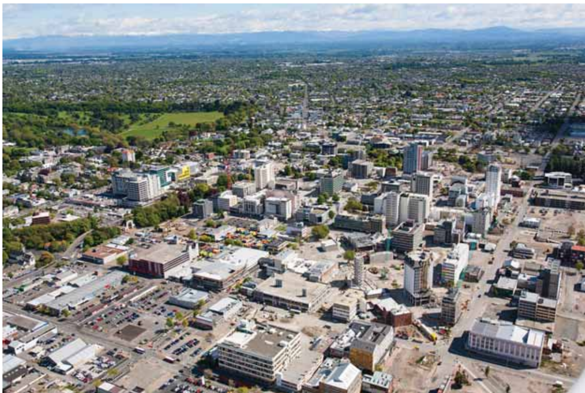
Figure 9: An aerial photo of Christchurch central city, October 2012, taken after many of the buildings had been demolished (source: Canterbury Earthquake Recovery Authority)
