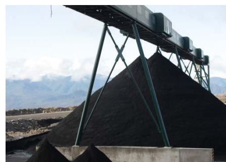
Stockton Coal Handling and Processing Plant.
