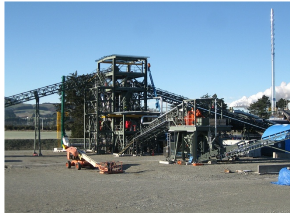
Construction of the Mataura Briquette plant
