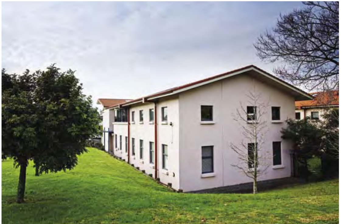
Above » Pitman House, Pt Chevalier, Auckland.
